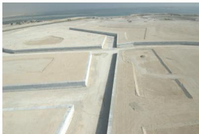
In order to overcome this problem the Contractor decided to perform part of the blue water dredging "in the dry". Complete working areas were closed off from the open sea via the construction of temporary bunds (in total 20 km). Fully confined areas were drained via the deployment 60 large dewatering pumps (of which 30 pieces with a minimum capacity of 3,000 m<sup>3</sup>/hr). The total set of pumps was able to dewater at a rate of approximately 100.000 m<sup>3</sup> per hour.
