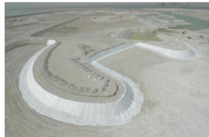
The total rock volume consisted of 2,5 million m<sup>3</sup> limestone and 4,5 million m<sup>3</sup> cap-rock. The limestone was mainly used as under layer for the shore protection whereas the cap-rock, after having been reduced to an acceptable size by means of crushers, was used as suitable fill in the reclamation.
